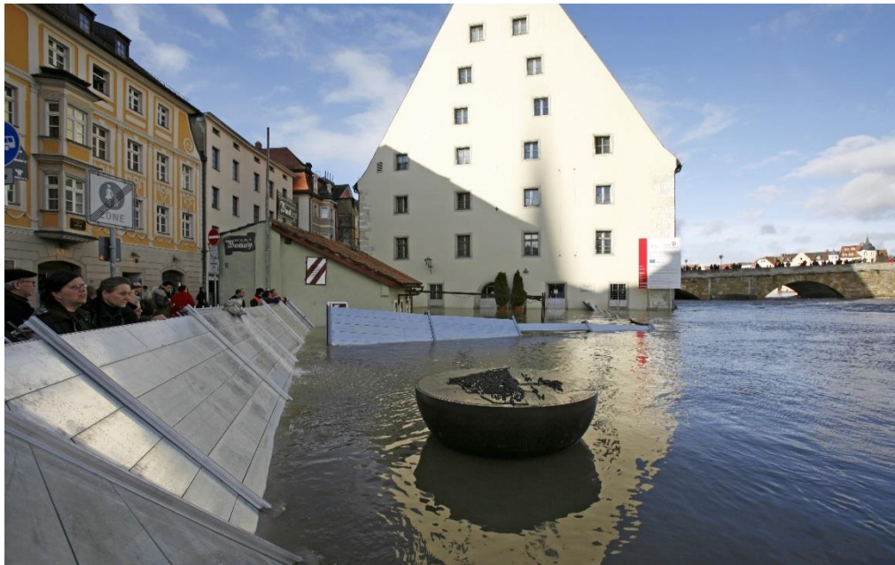
Figure 3. Mobile flooding protection in the area of the historic sausage kitchen / World Heritage Visitor Centre from 2013. © Bilddokumentation, Stadt Regensburg
