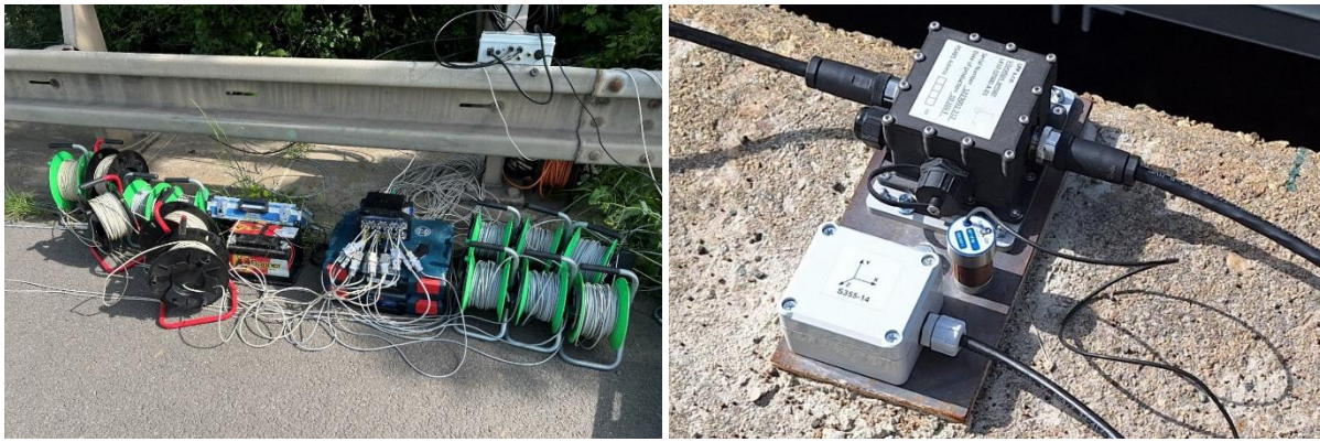
Figure 11: Bridge measurements: a) placement of measuring equipment, b) Seika B1 accelerometer
