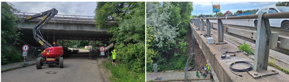
Figure 1: Bridge on Road I/50 in Brno: a) underside view, b) installation of measuring equipment”
