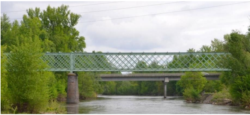
Figure 2: View of the second span of the bridge (P1-P2) from upstream
