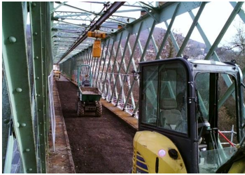
Figure 6: View of the dumper before demolition
