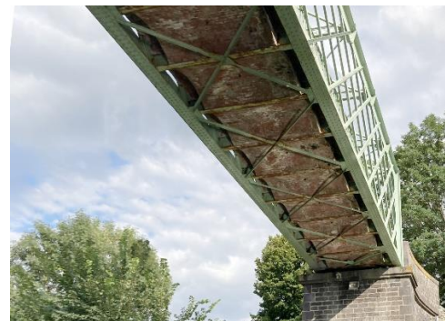
Figure 5: Bottom view of the existing bridge deck
