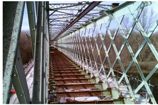
Figure 7: View after deck demolition
