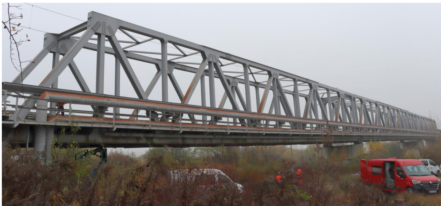
Figure 1: View of the bridge
