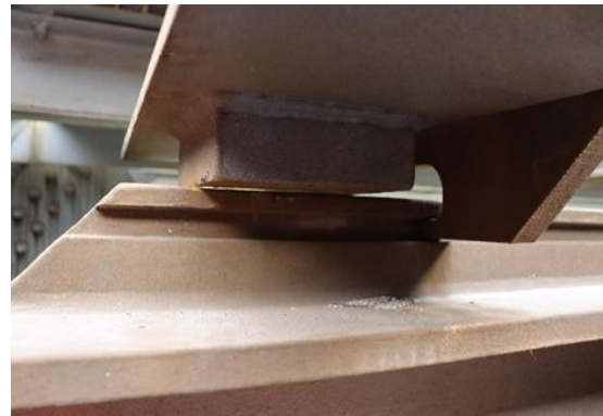
Figure 3: Installation of steel sleepers on the stringers
