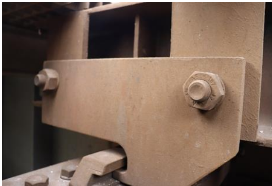
Figure 3: Installation of steel sleepers on the stringers
