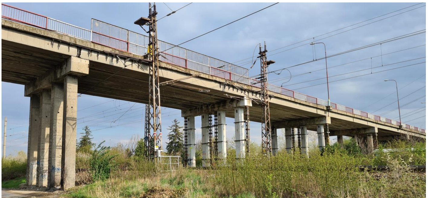
Figure 3: View of the bridge on Bojnicka Street
