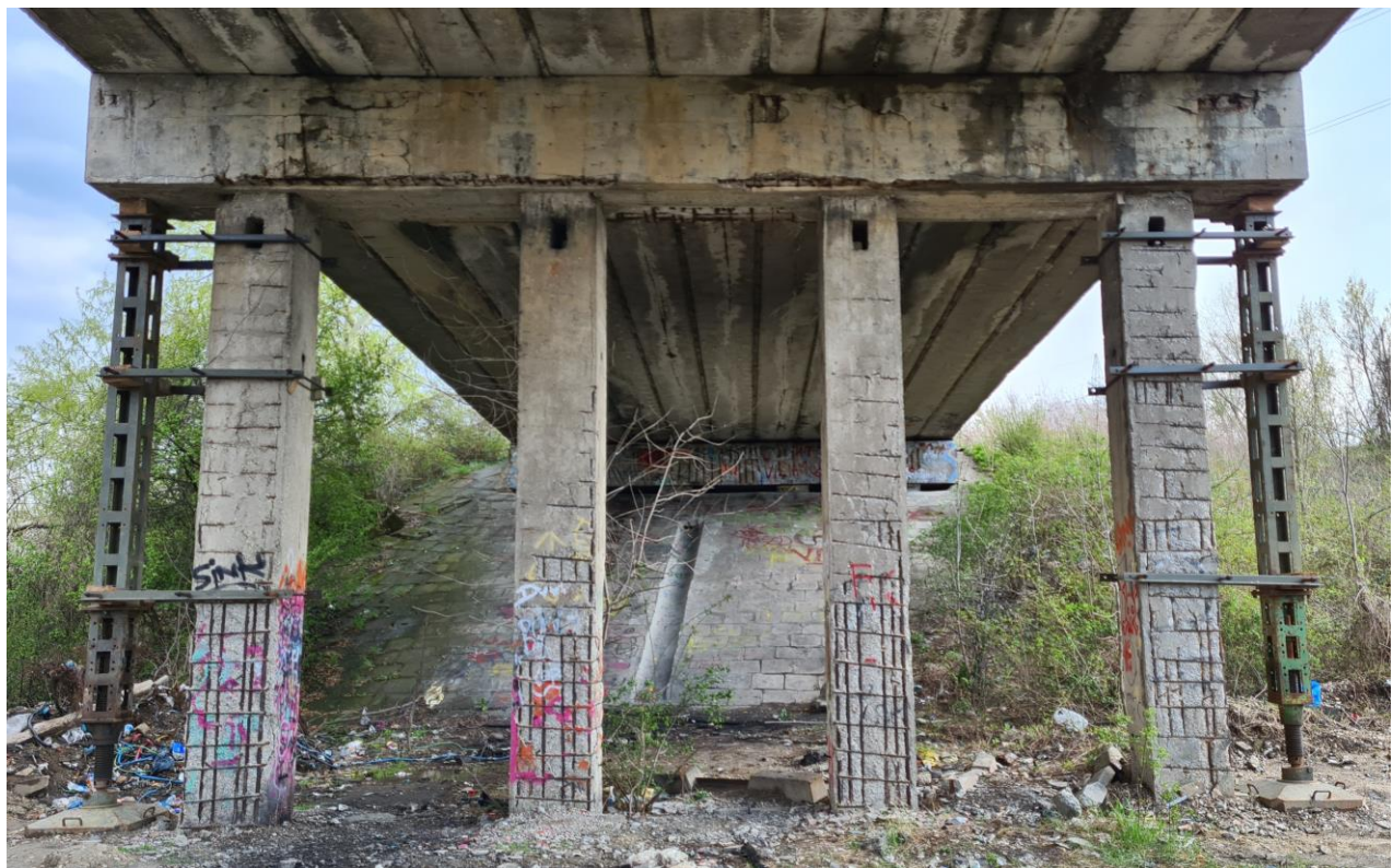
Figure 6: View on the substructure with temporary support of the crossbeam
