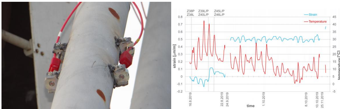
Figure 14: Strain-gauge measurement: a) installed vibrating-wire strain gauge, b) deformation and temperature record from a selected gauge
