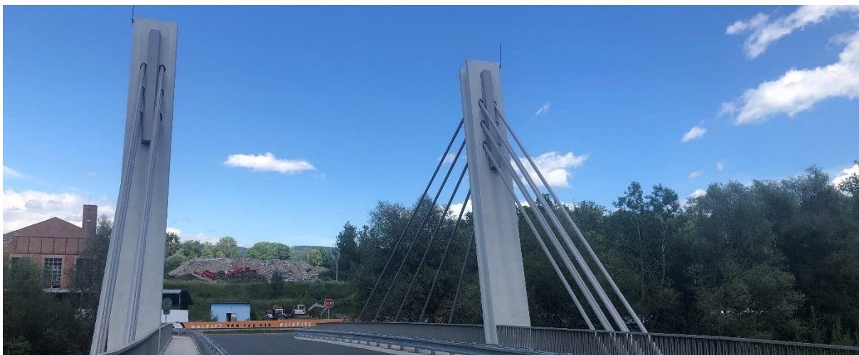
Figure 1: Cable-stayed bridge over the Rožnovská Bečva near Hrachovec
