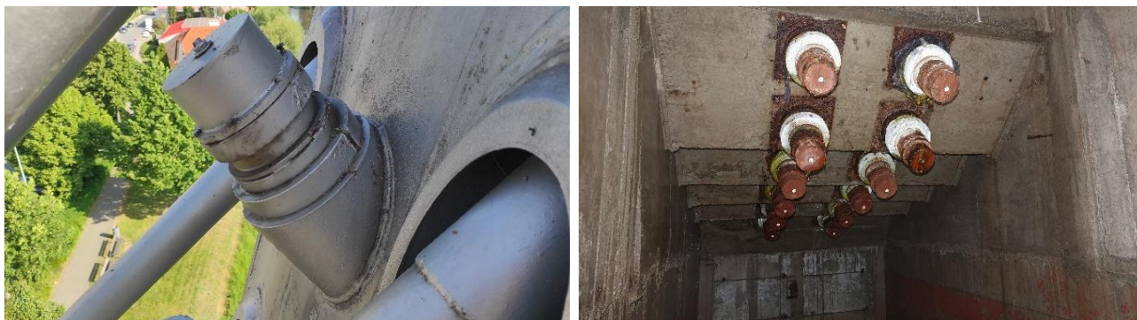
Figure 9: Condition of anchorages: a) on the pylon, b) in the anchorage chamber of the bridge over the Svatka River in Židlochovice
