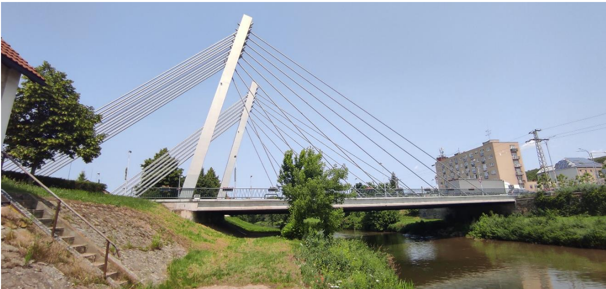
Figure 3: Cable-stayed bridge over the Svatka River in Židlochovice
