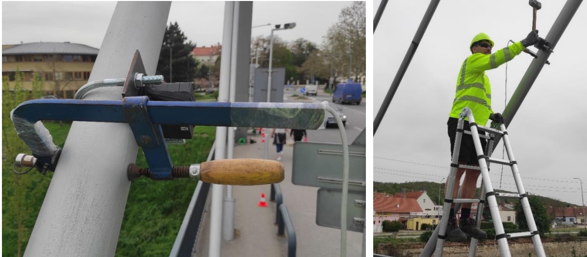
Figure 7: Conducting dynamic measurement: a) measuring fixture with mounted accelerometer, b) excitation by striking with a hammer fitted with a rubber head
