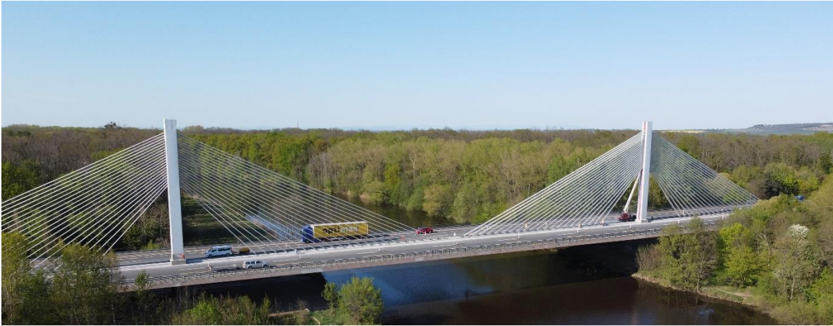
Figure 2: Cable-stayed bridge over the Elbe River near Poděbrady
