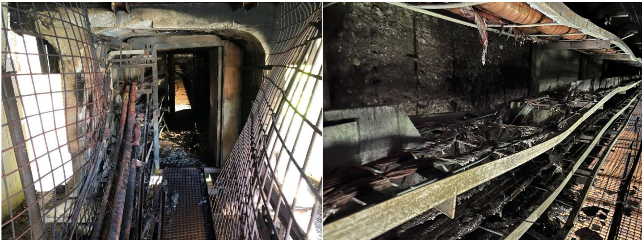
Figure 1: View at the entrance to the chamber of the footbridge and inside the chamber after the fire of the electrical cables
