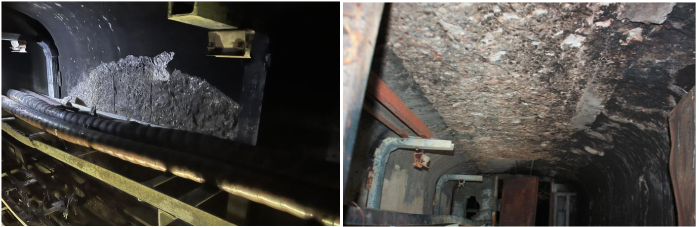
Figure 4: Spalling of the concrete inside footbridge box cell web on the left, RC slab right
