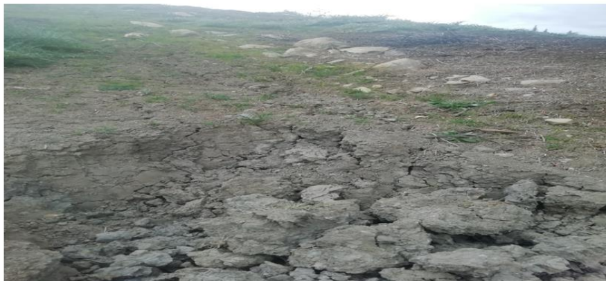
Figure 1: Surface shrinkage cracks in clay soil
