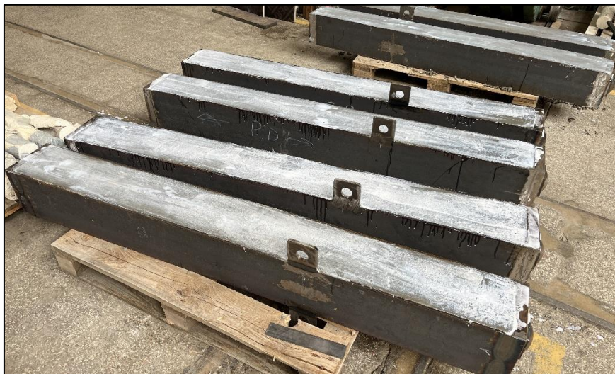
Fig. 6: Composite steel-concrete columns after casting of the concrete infill.
