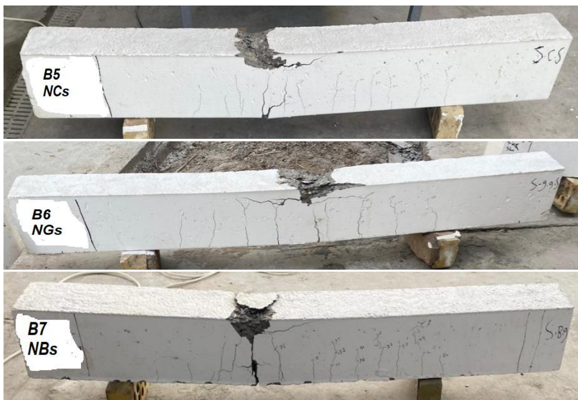
Fig. 6: Cracks pattern for NCs, NGs and NBs.
