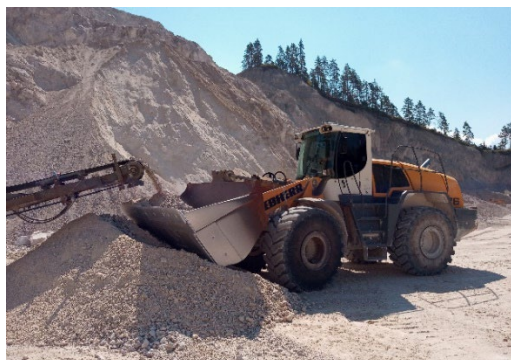
Fig. 5: Sorting and loading of the crushed aggregate fr. 0/31.5 mm in the quarry.
