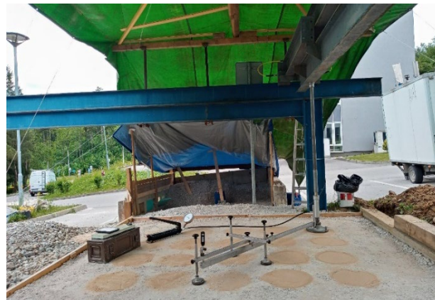
Fig. 6: Static load tests conducted on the surface of the last partial structural layer of crushed aggregate fr. 0/31.5 mm.
