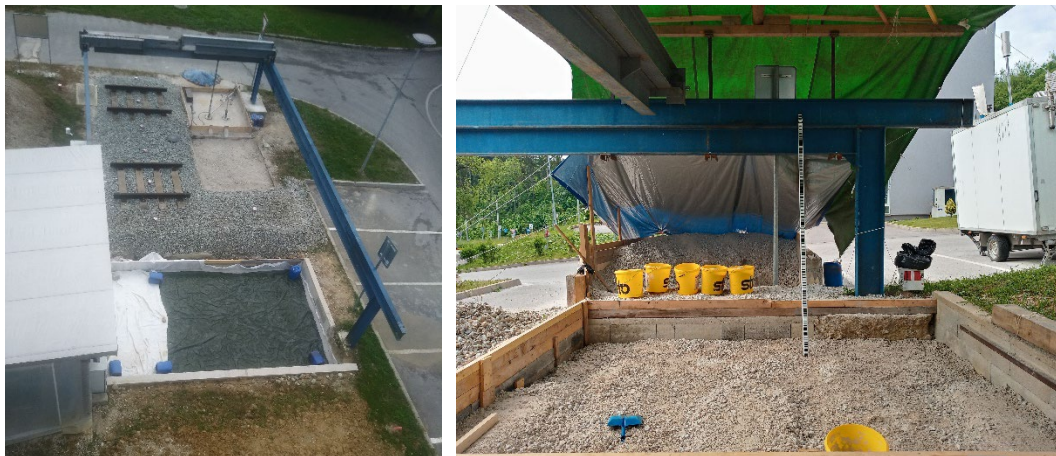
Fig. 1: Sector for assessing the deformation characteristics of building materials (left) and construction of the structural layer of the experimental field (right).
