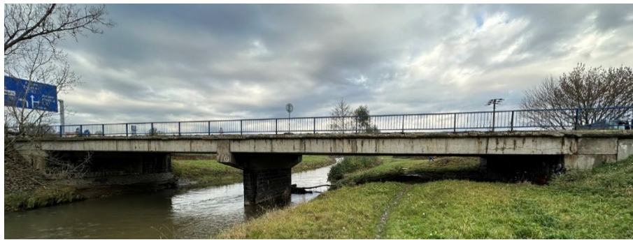
Fig. 11: Sideview on the Bridge "D" in Rimavska Sobota.
