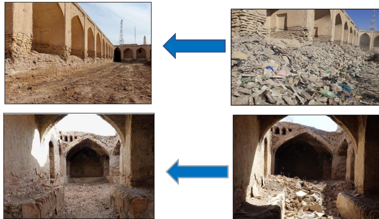
Figure 12. Pictures showing preventive measures (removing roof rubble) (survey photos in 2023 by researcher)
