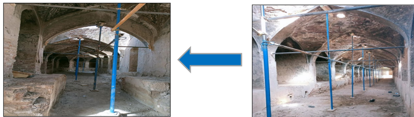
Figure 13. Pictures showing preventive measures (Supporting walls and ceilings) (survey photos in 2023 by researcher)
