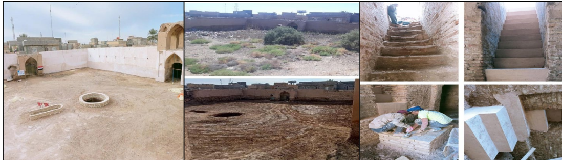
Figure 16. Pictures showing preventive measures (Cleaning wells, removing dust, and repairing stairs) [21]
