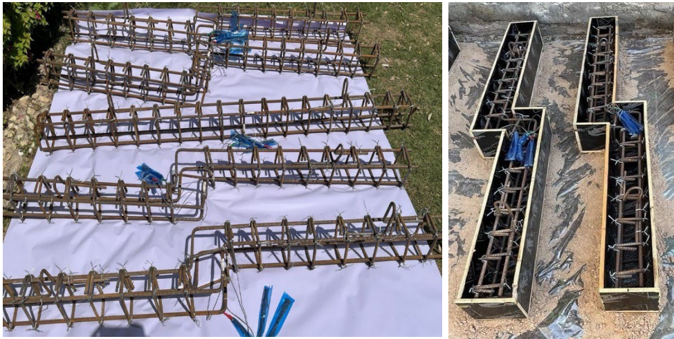
Fig.4 The steel reinforcement in the farmwork.
