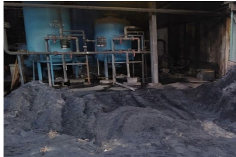
Fig. 1: The POFA is disposed of beside the Boiler furnace.
