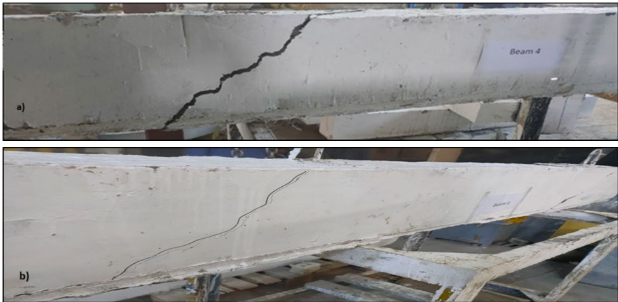
Fig. 15 Cracks Pattern in Beam BSSFT a) left side, b) right side
