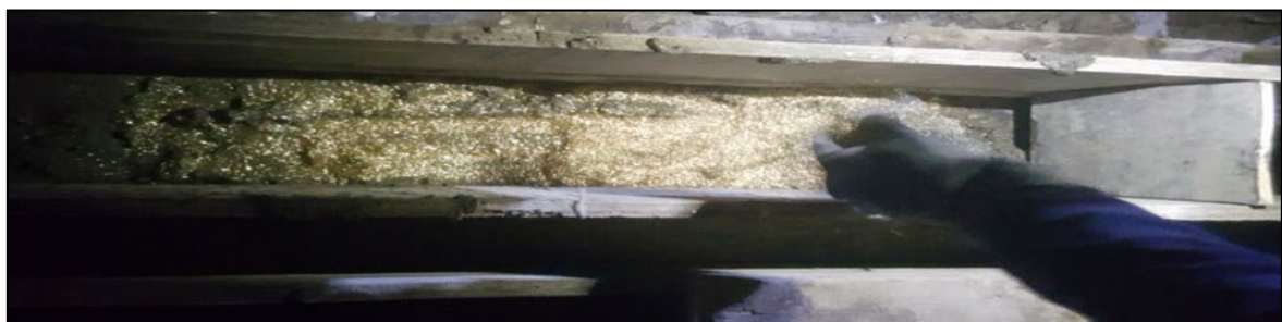
Fig. 3: Casting the Strengthening Beams
