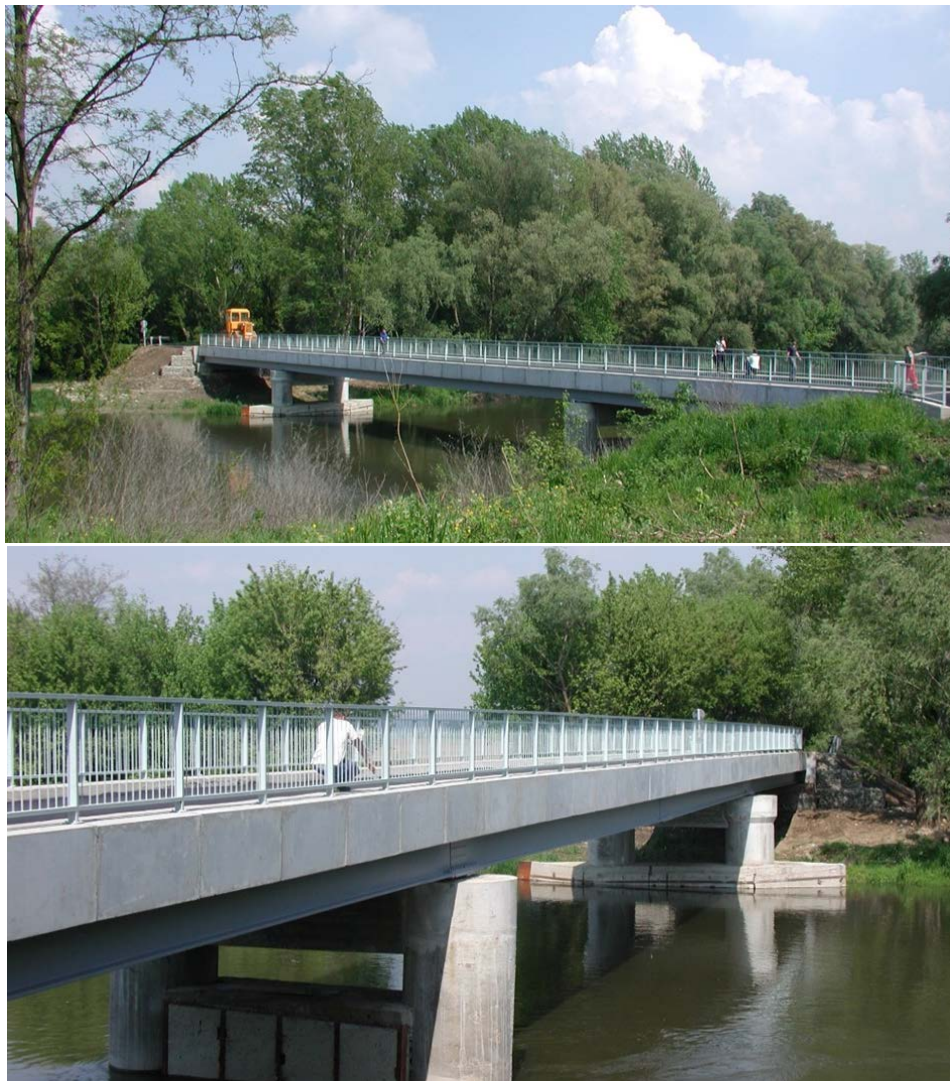
Fig. 7: Views of the reconstructed bridge.
