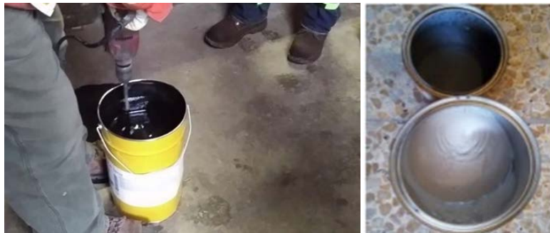
Fig. 6: Mixing of Sikadure-330.
