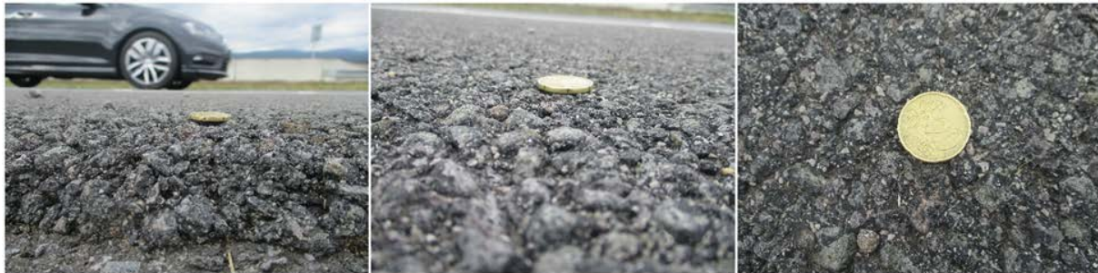
Fig. 5: Views of SMA O 11 using CRM asphalt.
