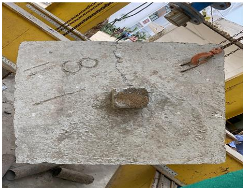
Fig. 18: Yield line crack pattern of voided flat slab (Initial crack).
