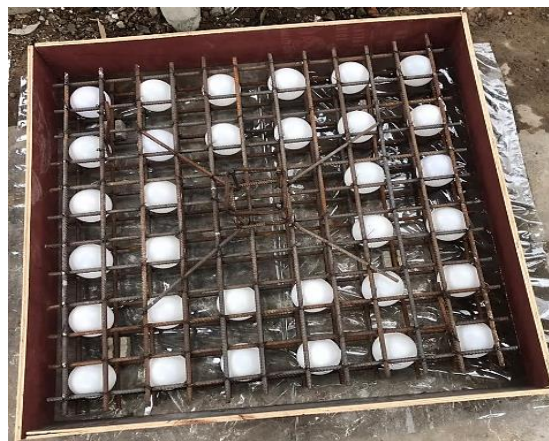
Fig. 2: Actual photograph of voided flat slab in the mould.
