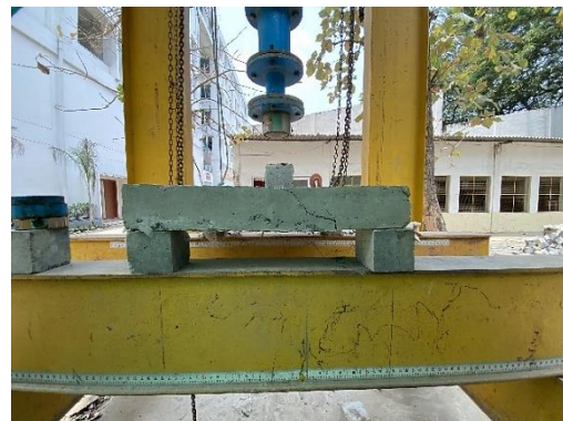
Fig. 21: Yield line crack pattern of voided flat slab (36VS6).
