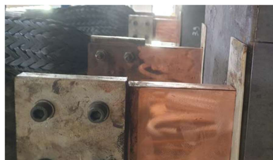
Figure 6. System for clamping the copper bars in the supporting bracket
