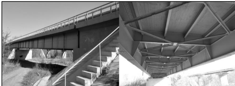
Fig. 1 – Real life view of the Mircești Bridge over Siret River.
