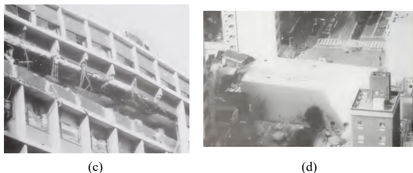
Fig. 9 – (a) “Second story collapse – commercial building in downtown Kobe; (b) Third story collapse – Downtown Kobe; (c) Upper story collapse – Downtown Kobe; (d) Totally collapsed building on Flower Road” (NIST Special Publication 901, 1996).
