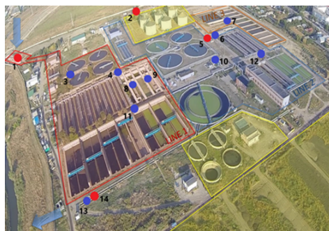
Fig. 3 – The study area - Iași WWTP.
