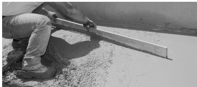
Fig. 1 – Leveling screed made with cement, sand and water ( https://www.betonexpert.ro/sapa-de-egalizare ).
