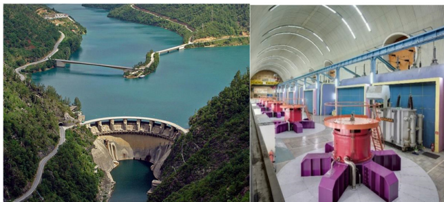
Figure 1: Dam and HPP Jablanica
