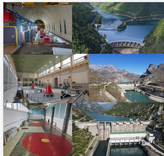
Figure 6: Cascading series of HPP on the Neretva River basin (up); HPP Jablanica, Grabovica and Salakovac (down).
