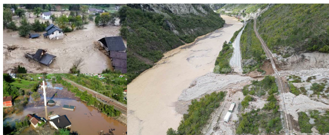
Figure 9: Landslides recorded on the M-17 road (Komadinovo vrelo, Prenjska vrata, Donja Jablanica)
