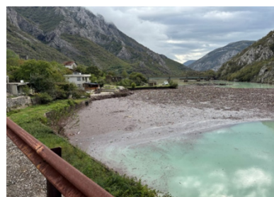
Figure 10: Waste came to the surface of the reservoir and nearby dams
