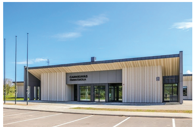
Fig. 12. Modular-type buildings for temporary operations at Carnikava Primary School [38].
