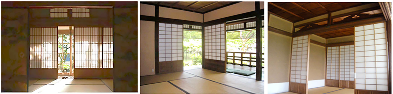
Fig. 13. Use of washi paper in traditional Japanese architecture [9], [26].
