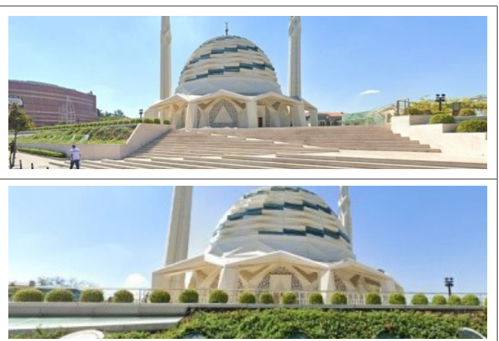
Fig. 24. Road facades of the Marmara İlahiyat Mosque [48].
