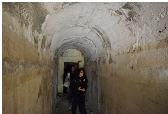
Figure 11 Interior spaces of the Underground "City" of Kukës
