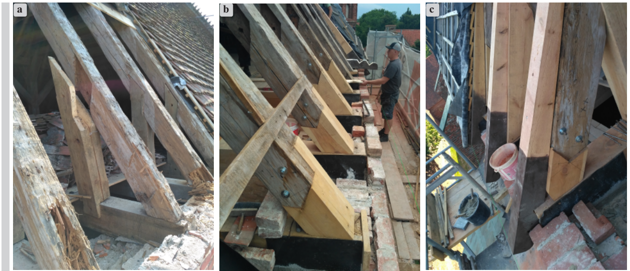
Figure 4. The eaves zone of the roof a) damaged ends of rafters and floor beams; b) repaired rafter ends; c) correction of the eaves' length by the use of chantlates
