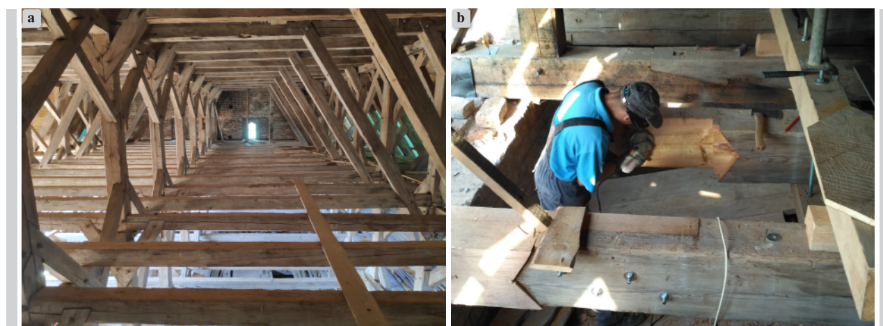
Figure 3. The internal part of roof truss a), structural elements, b) work on replacing the beam
