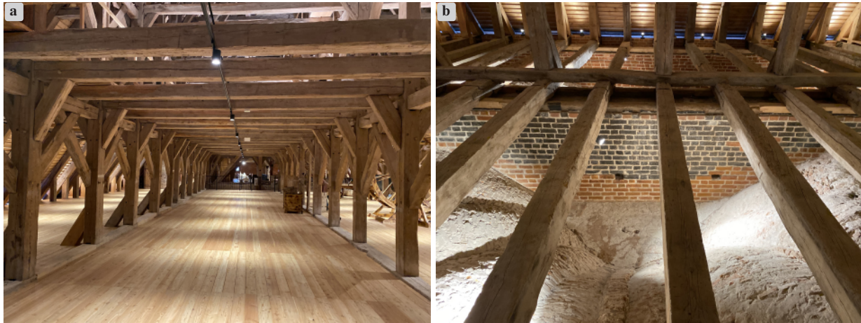
Figure 7. The attic space after renovation a), roof truss and wooden floor; b) vaults over the nave
