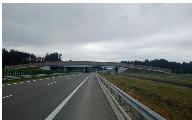
Fig. 2. Properly planned and implemented game crossings partially eliminate the negative impact of road infrastructure on the functioning of the population Source: own elaboration.
